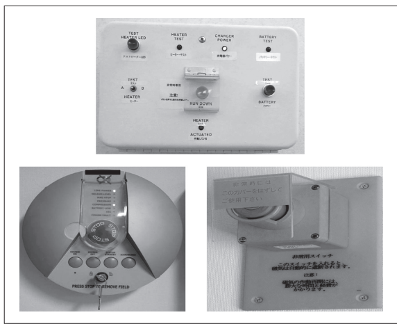
Fig.1 Various kinds of quench buttons The structure and colors is different among the MR manufactures.
